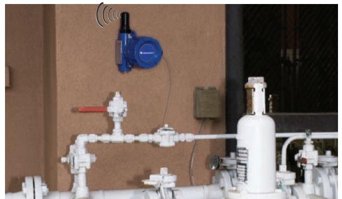
UWXL , long range wireless transmitter, connected to an RTD used to monitor surface temperatures remotely. Visit newportUS.com/uwxl
