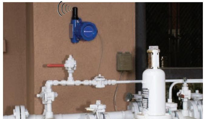
**UWXL**, long range wireless transmitter, connected to an RTD used to monitor surface temperatures remotely. Visit [newportUS.com/uwxl](http://newportUS.com/uwxl)
